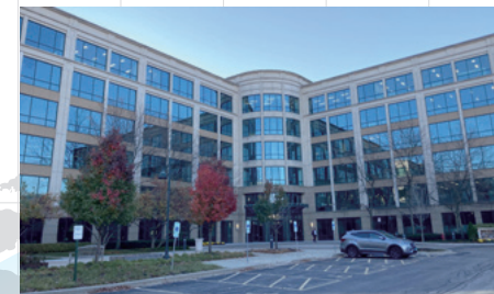
Office building to which we will be relocating
